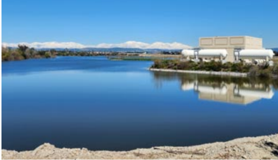
The Orange County Groundwater Basin, managed by OCWD, continues to provide a local, reliable water supply for 2.5 million people in north and central Orange County.
